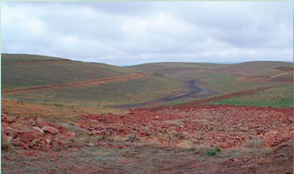
Long, constant-gradient slopes • Gradient Terraces Rip-rapped drains
